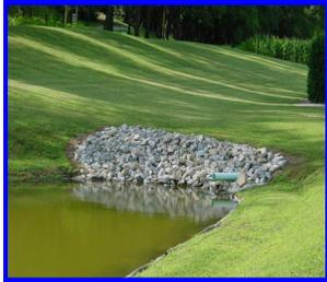
**Outlet Pipes** direct storm water from a detention pond to a nearby creek or stream. Typically, there is only one outlet associated with a pond. The outlet may consist of a single pipe, a riser pipe, or some other overflow structure.
